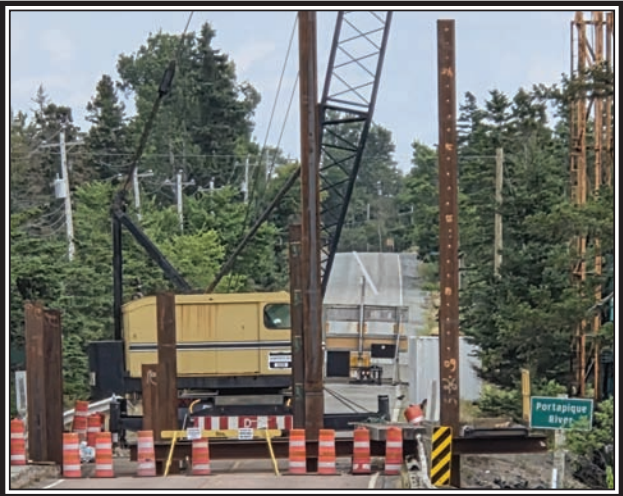
This recent weekend photo shows the pilings in recent depths of driven into the river bed at the Portapique Bridge awaiting return of the construction crew. Many had expected the bridge to open at the end of August, but it will be well into fall before the bridge reopens. (Rees Photo)
