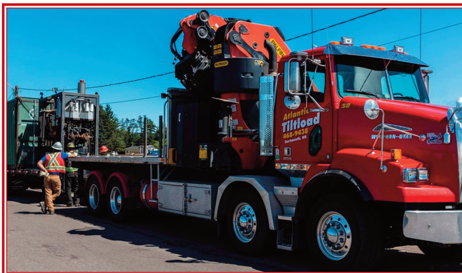
Atlantic Tiltload equipment was used to remove equipment from the R J MacIsaac Construction barge in Parrsboro on August 19th and delivered to another barge owned by MacIsaac's in Sheet Harbour. (Lawrence R. Nicoll Photo)
