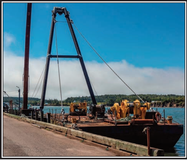
The R J MacIsaac Construction barge has been a part of the scene at the Parrsboro Wharf since the company laid the sub-sea data lines on the FORCE Site. (Lawrence R. Nicoll Photo)
