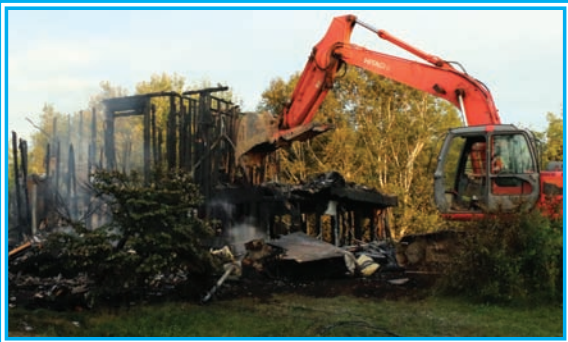
An excavator was brought in to knock down the remaining structure so fire fighters could put out any remaining hot spots.
