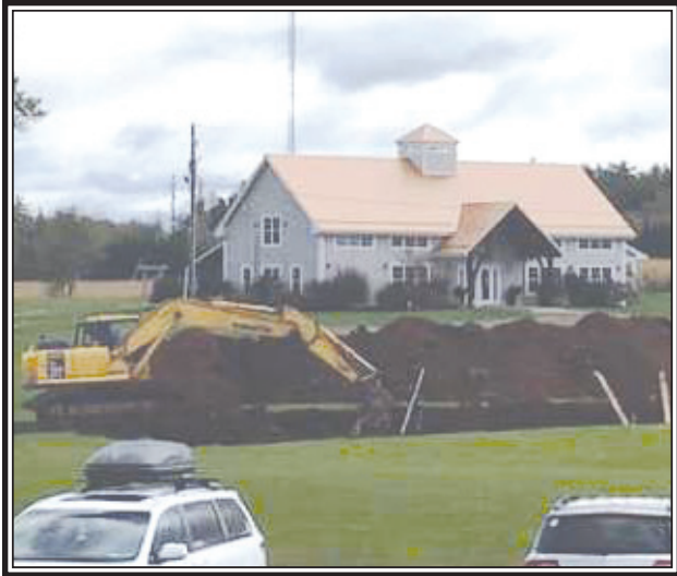
Ground was broken for the new Pharmacy in September 2019.
