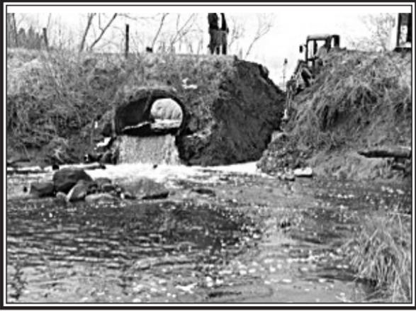
Mike Parker (East Coast Aquatics) digging the trench to hold the Steep Pass Denil. The denil was inserted separately from the pre-existing culvert to prevent any damage. (Submitted)
