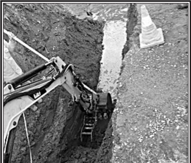
Sediment and soil being removed to place the denil structure in place. (Submitted)
