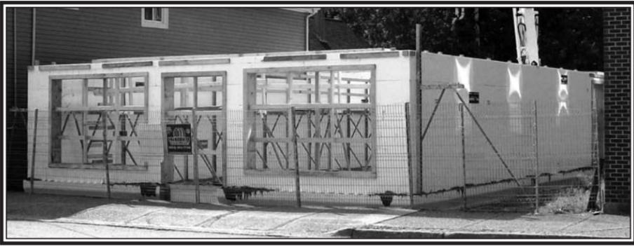
Construction of the new home for Colchester Food Bank has started. The Insulated Forming System (ICFS) walls – insulation which is filled with concrete will provide an energy efficient building. Construction is expected to be completed by late fall. (D Brown Photo)
