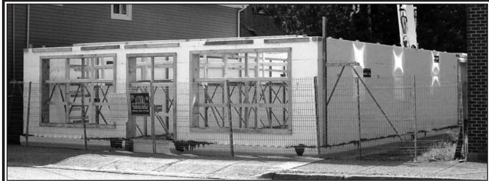
Construction of the new home for Colchester Food Bank has started. The Insulated Forming System (ICFS) walls – insulation which is filled with concrete will provide an energy efficient building. Construction is expected to be completed by late fall. (D Brown Photo)
