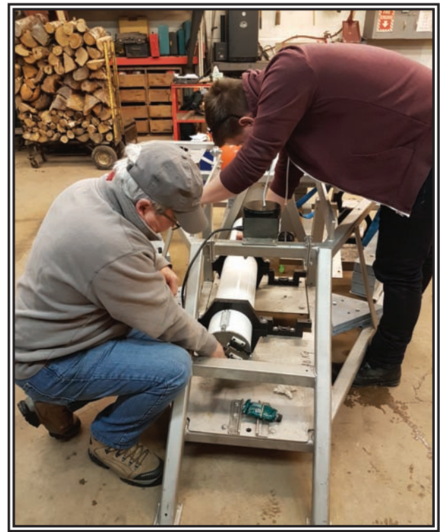
Murray Scotney (OceanMoor Technical Services) and Tyler Boucher (FORCE ocean technologist) install the acoustic zooplankton and fish profiler on the FAST-3 underwater sensor platform.
