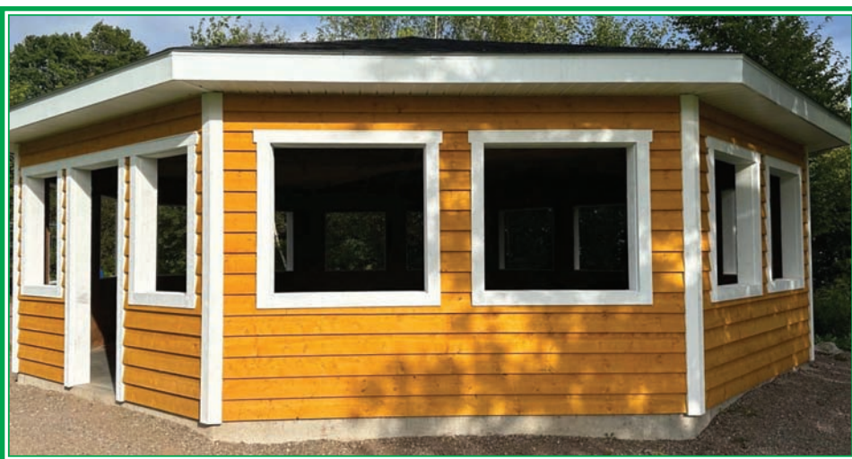
Masstown Market graciously provided the materials for the construction of the outdoor classroom, which was built in Phase 2, thanks to Dan MacKay Construction and Tidal View Construction.
