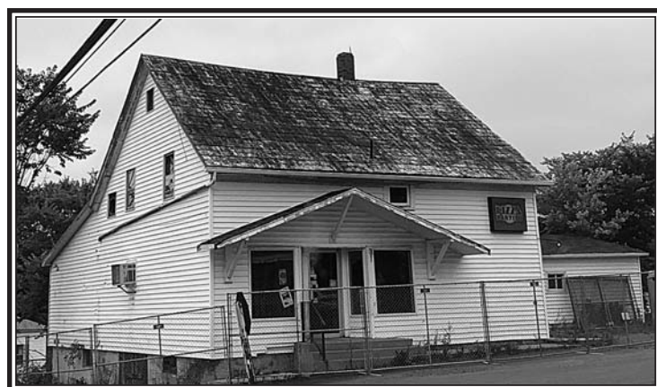
The iconic Barnhill's Store, Debert is going to be demolished by Dept of Transportation. It is not known why NSTIR wanted the property. (Harrington Photo)
