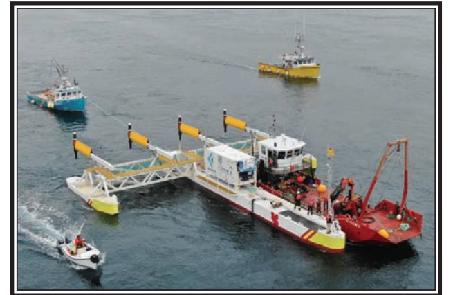
The PLAT-I platform with the installation flotilla made up of Kipawo (Huntley's Sub Aqua Construction) TyKiSha-J (Westport) Island Lady G (Freeport) and Puffin (Luna Ocean Consulting) during installation operations in Grand Passage. (Submitted)
