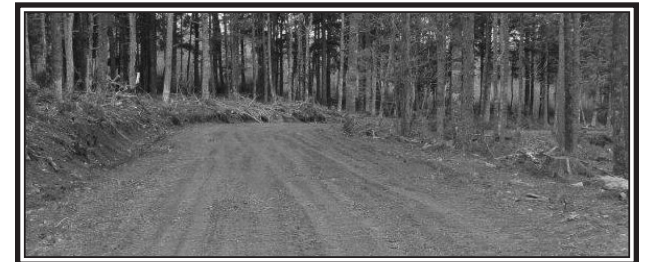
Some roads have been built to help get product to roadside and provide easier access for forest management. (Submitted)
