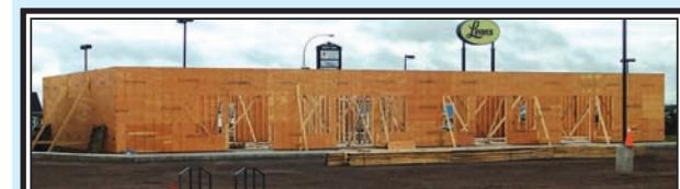
Referred to as Building #3 in the Truro Power Centre new mini-mall, this side walls are up and the roof trusses are on-site and will be installed soon. (Rees Photo)
