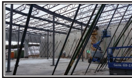
The East Coast International building at Truro Power Centre was built with insulated pre-cast concrete panel walls supplied by Eastern Structural Pre-Cast Ltd, Milford plant. This photo shows the panels braced to hold into position until secured to the building's structural frame. Workers can be seen completing the installation. (Submitted)
