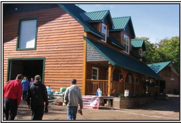
The new sugar shack occupies approximately one third of the new building which also incorporates the Harrison family's home. In-floor heating from a propane source makes it comfortable for the family and workers during the maple season. (Rees Photo)
