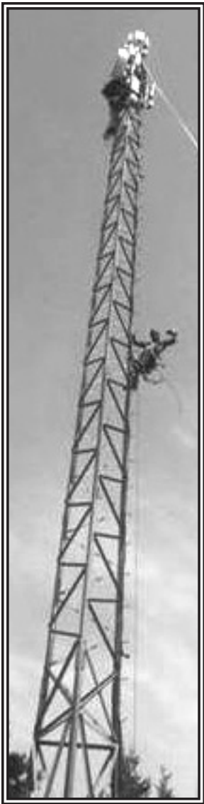
Workers climb up a Seaside Tower to install new equipment.
