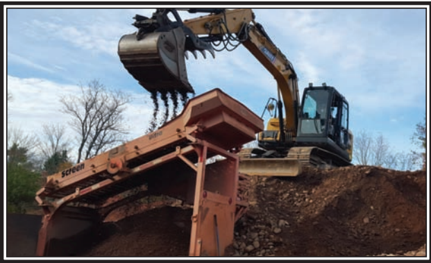
Don Turner runs the screening plant every day unless the boys need a load of gravel.
