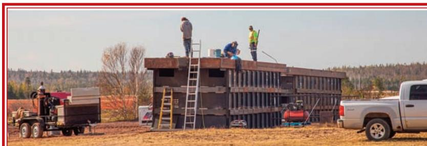
Four RR Ore cars appeared in Parrsboro at the Harbour on the local property. The cars are going to be filled with cement and used as anchors for the new tidal turbine. Currently, they are on land near the furnace factory with flat portions being welded. (Lawrence R Nicoll Photo)
