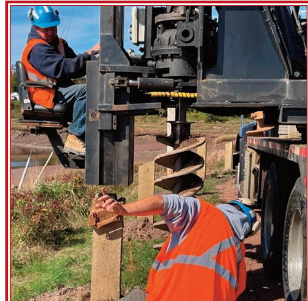
Workers with Eastern Fence Erectors line up a new guardrail being installed on Two Islands Road in Parrsboro.
