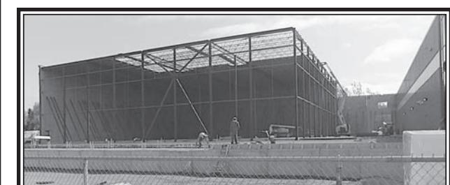
Tradesmen installing exterior sheathing and roof of a large addition to the Tim Hortons Depot in Debert on September 25th. (Rees Photo)
