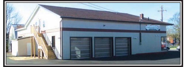
The three automotive bays in the main building can accommodate larger vehicles. (Rees Photo)
