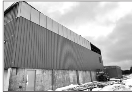
The back wall is currently being repaired on the tipping floor building where panels blew off. The thermal camera that was on the back wall has now been put back in place and is operational again. (Contributed)
