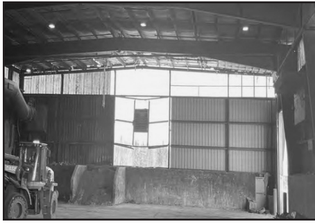
The back wall is currently being repaired on the tipping floor building where panels blew off. The thermal camera that was on the back wall has now been put back in place and is operational again. (Contributed)
