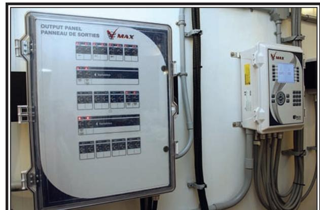
The GSI Electronics V-Max for ventilation, lighting and run times for egg belts and feeding was supplied by Eric Griffin Agriculture Equipment Ltd. of Kentville.
