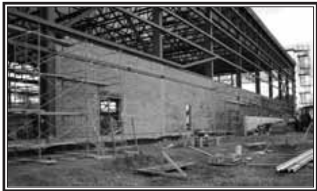
Concrete block goes up on the arena side of the facility, facing MacClure's Mills Rd.
