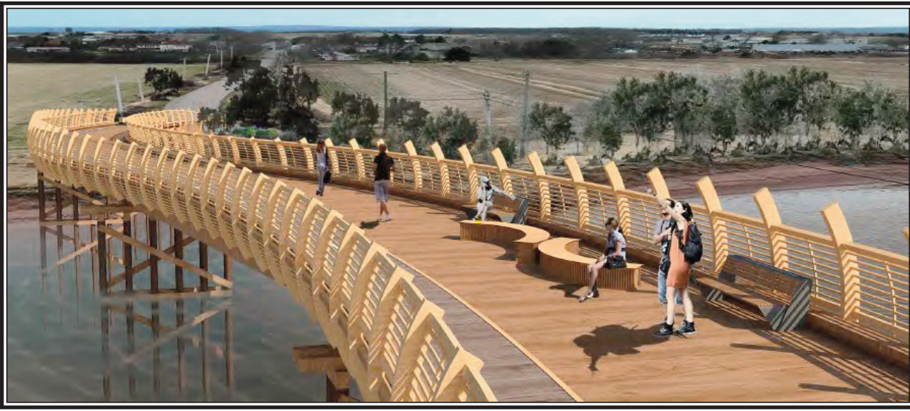
WRD & TRS: Price: $7,901.019. Completion Date: January 2027 Design: Glulam girder-under bridge. Span: 130m supported by three timber "in water" piers
