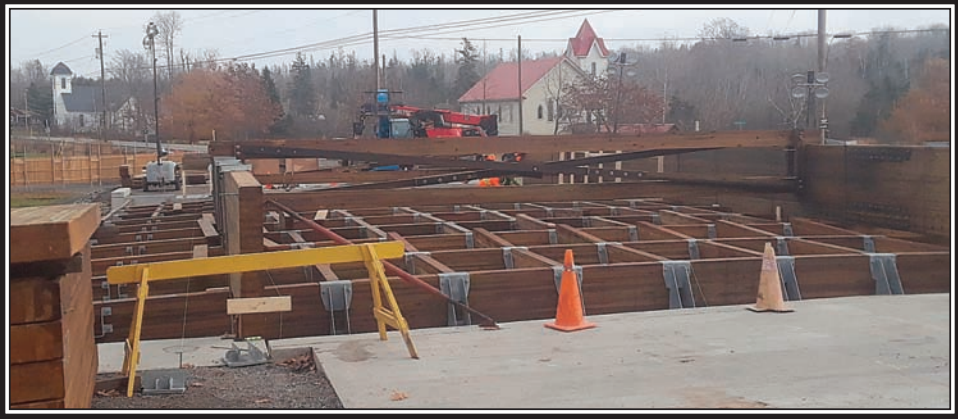
The deck super structure for the Bass River bridge sits idle on January 28th. Work on the bridge will start in April after the road closure season is over and asphalt plants have re-opened. (Rees Photo)
