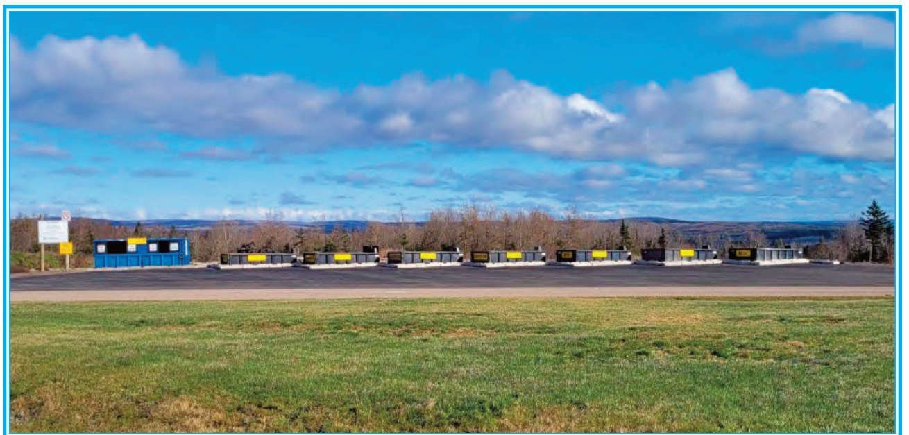
As shown above the public drop off redesign at the Kemptown material handling facility is now complete and operational. Philip Reddin told council on February 13th. "We have received positive feedback from customers as it has much more space for traffic flow and has a more secure location behind our gates". Mr. Reddin's additional reports are found on pages 10, 11 and 14. (Colchester Photo)
