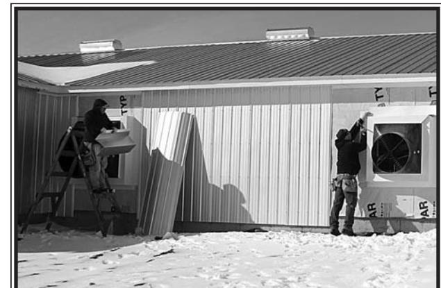
Contractor Clint Verheul has been busy working on the expansion at Bayview Poultry Farm. Ventilation fans are being installed in the new laying barn.
