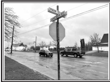
The Municipality of Cumberland has awarded Dexter Construction Company Ltd. the contract for the Junction Road Rehabilitation Project for a value of $7.292 million plus HST. Darrell Cole – Municipality of Cumberland
