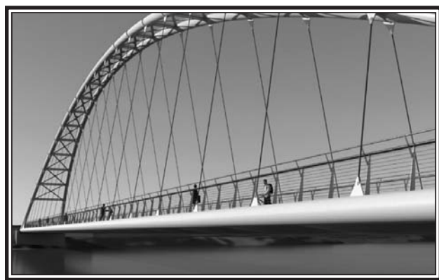
This artist conception shows a portion of the side with pedestrians on the deck, with the cables and the basket handle arch. (Submitted)
