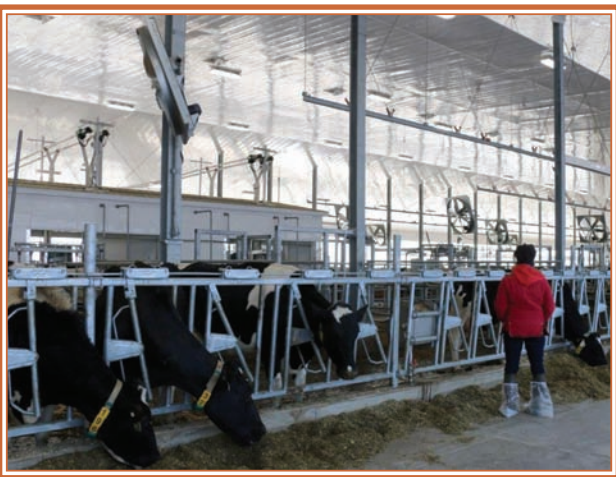
Automated fans keep the temperature controlled for cow comfort.
