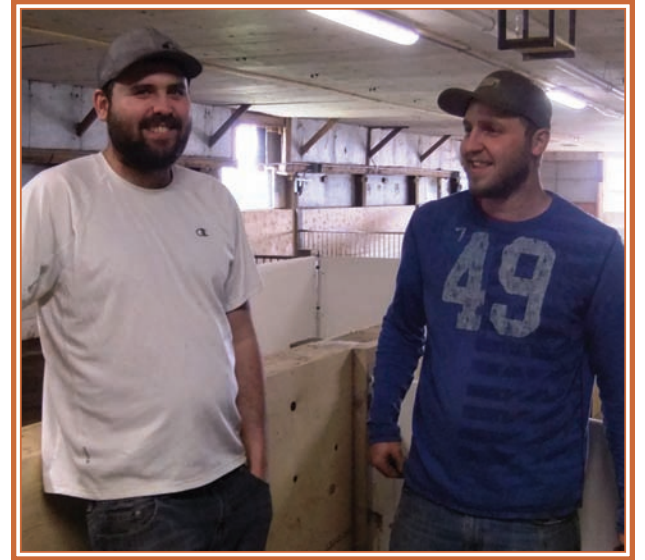
Brandon & Jonathan Millen shown in the partially renovated hog barn on the Meredith Farm, where they expect to raise approximately 500-600 pigs per year, with most of them going to the new butcher shop at Masstown Market. Water lines and automatic feeders were installed as the hog facility was being updated. Story and more photos on page C5. (Rees Photo)
