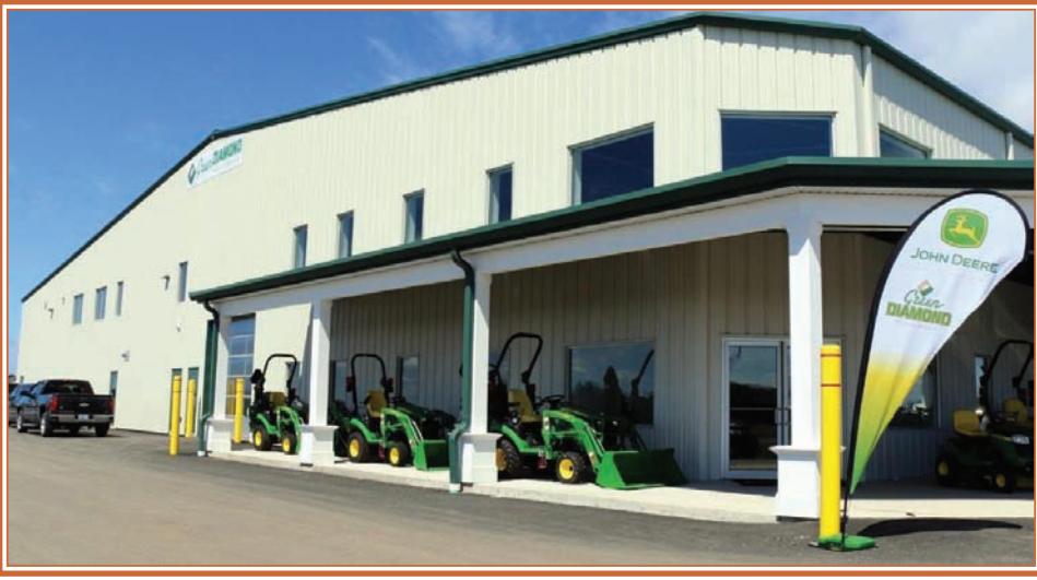
The new 56,500 square-foot Green Diamond Equipment Ltd. location at Hub Drive, Upper Onslow.
