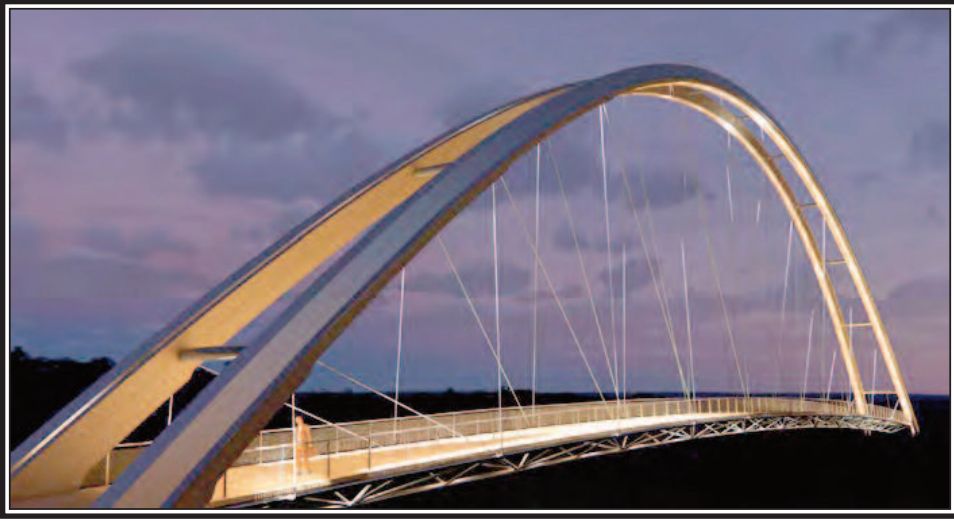
Balodis & Structure Craft: Price: $13,500,000 Completion Date: October 2026 Design: Parabolic Arch – Glulam & Prestressed Timber Deck Span: 120m full span
