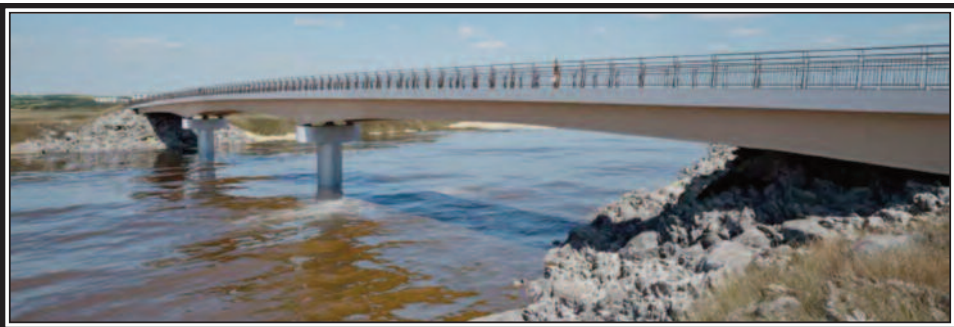
Pomerleau & EXP: Price: $13,420,308 Completion Date: November 2026 Design: Double “I” Beam. Span: 130m supported by two “in water” piers.
