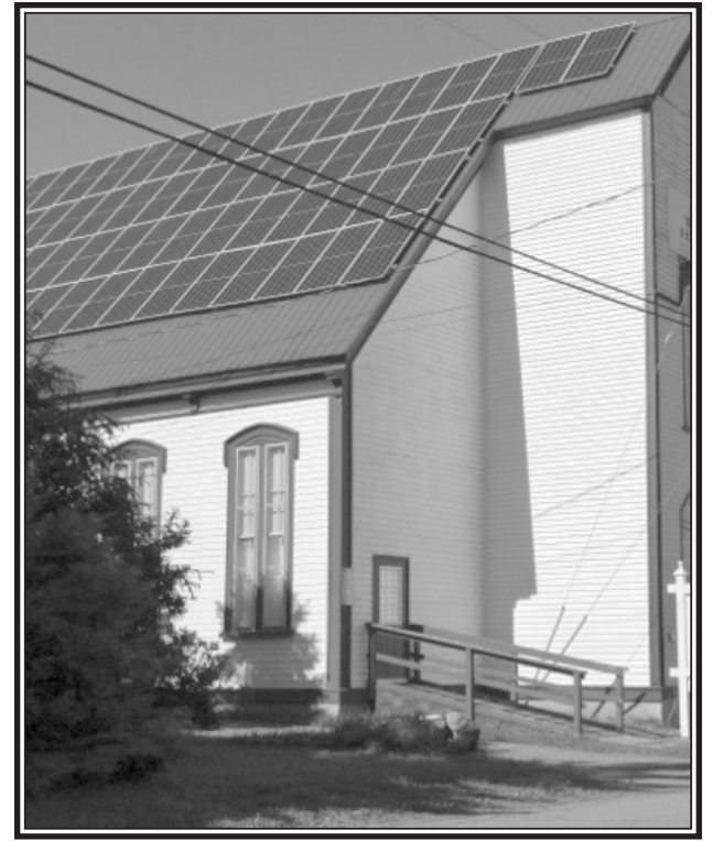
The hall showing Solar panels. (David Townsend Photo)
