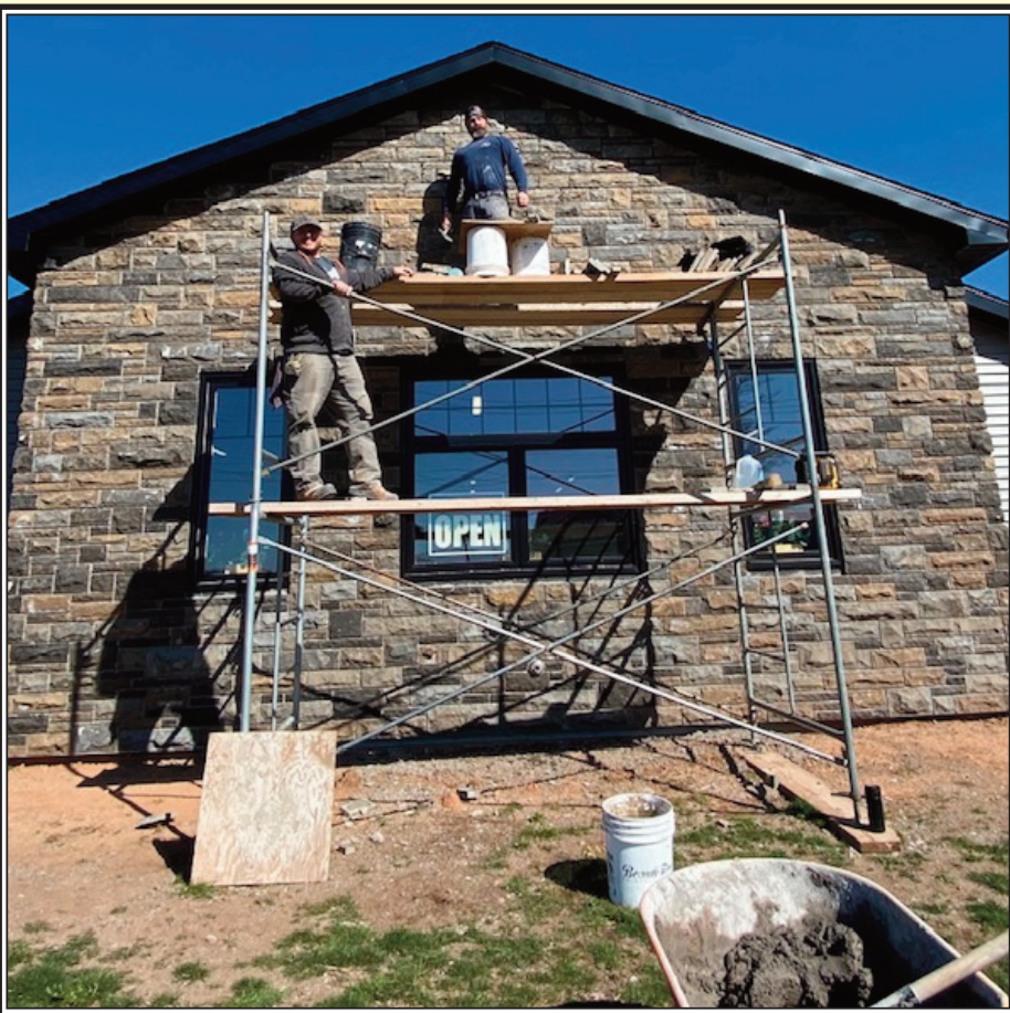
An open sign adorns the showroom window even though tradespeople are completing installation of the exterior siding. (Submitted)
