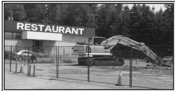
There's been plenty of excavation activity at the Double C Truckstop recently as Imperial Oil removed and treats contaminated soil from the site of previous diesel tanks. Next will be removal of contaminated soil from the gasoline tanks from years gone by. (Rees Photo)
