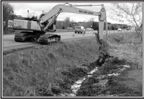
The Ditch Doctor at work along junction of Hwy #2 and #4 near the Masttown Market. The Ditch Digger head, made by Adam Fisher, provides a more environmentally friendly way to clean out a ditch, with a much smaller channel and less erosion to surrounding banks. A video of the machine at work can be viewed at online at [www.youtube.com/watch?v=Dz7A\\_47SfNk](http://www.youtube.com/watch?v=Dz7A_47SfNk) (Harrington Photo)
