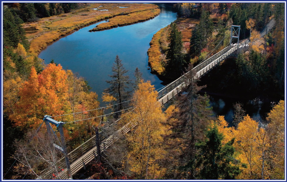
The new suspension bridge is located on the Ketchum Trail and replaces the original bridge that opened in 1996. Antony Spalton photo.
