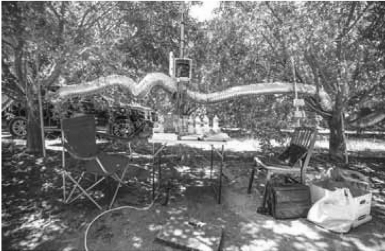
Exhaust from a propane generator and several vehicles is collected and fans funnel it through a system of ducts. The cooling system uses water from a children's pool, a pump, a sprinkler and a condenser.
