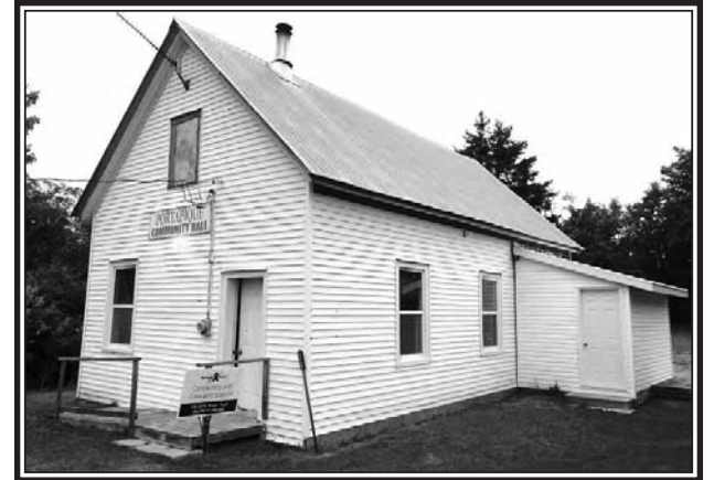
Portapique's Riverside Community Hall
