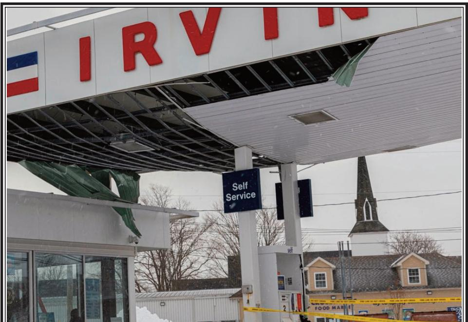
Friday's storm damaged the underside of the large exterior canopy at Leigh Wheaton's Irving. Note the missing underneath portion of the sign. Yellow caution tape was strung around the pumps, directly under the portion of the canopy which remained loosely in place. (Lawrence R. Nicoll Photo)
