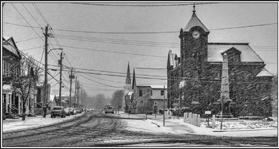
Framed by the old post office, Parrsboro's Main Street is always a scenic beauty even during the height of howling winds blowing the snow around.
