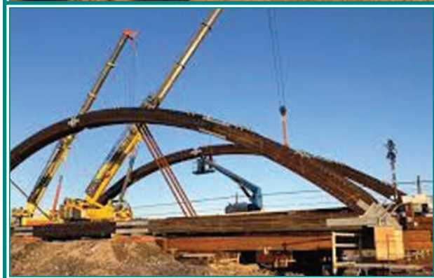
Cranes have completed installation the exterior arches and putting the deck in position. (Google Images) Insets: Built at a cost of $3-Million the new wooden Nappan bridge superstructure, to be named after Roger Bacon, is ready for the decking. (Google Images) (Google Images)
