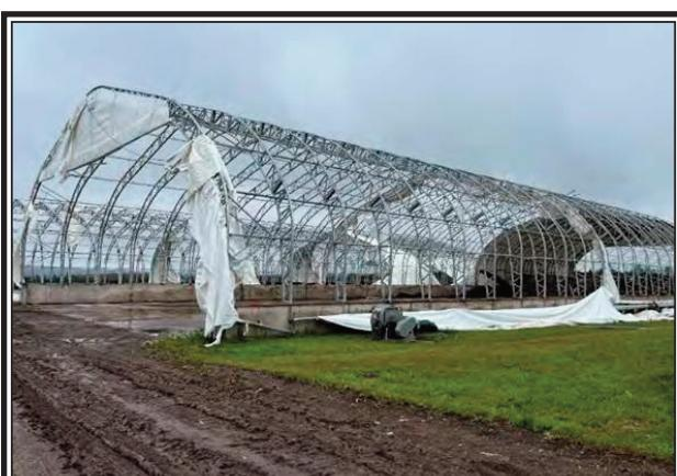
All three of the Compost Megadome structures were damaged in the hurricane. Manufactured by supplier, Megadome, was in the week after the storm to secure the framework and remove the tarps or hanging metal so that the buildings could be put back into use while awaiting repairs. The municipality hope to have 1-2 of the tents repaired before the end of the year. (Redden Photo)
