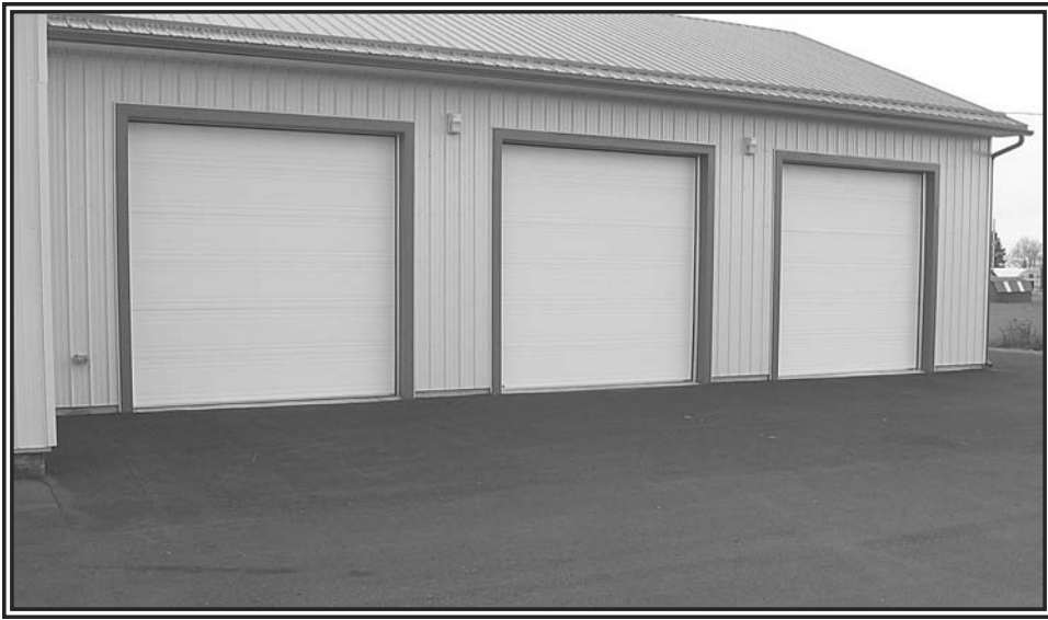
Not only is the parking area of the new addition to the Economy Fire Hall sporting a fresh look, the area in front of the original hall also received driveway sealing thanks to a special gift from Vernon Wamboldt. In mid-October, Wamboldt who operates Vern's Driveway Sealing applied his product to the paved areas, free of charge to benefit the community. He did it in memory of George Faulkner. Within a couple of months we'll have a special detailed story on the history of how the firehall was built at this location. The research is being done now. (Rees Photo)
