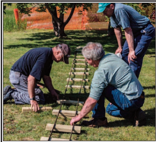
It took many hours to lay the precisely lay the track for the weekend. (Lawrence R. Nicoll Photo)
