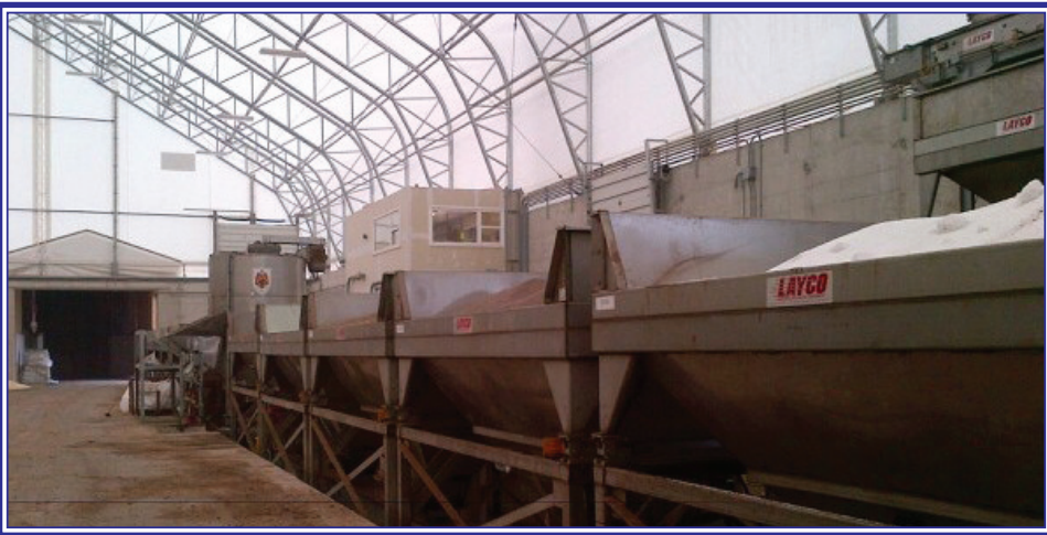
This photo shows part of the interior of the Truro Agromart fertilizer plant that was built in 2015. (Submitted)
