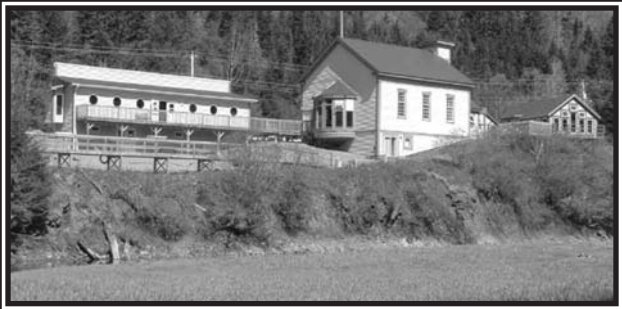
In 20 years the Age of Sail Heritage Centre and Museum have become an identifiable landmark as seen from the river.
