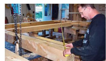
All of the layout and cutting of the more complex joints is done on the sawhorses at once. It may take 20 minutes to carve a nice tenon for that mortise, ready for a wooden peg to be tapped in on the big day of the raising. We leave the screw guns for the drywallers.
